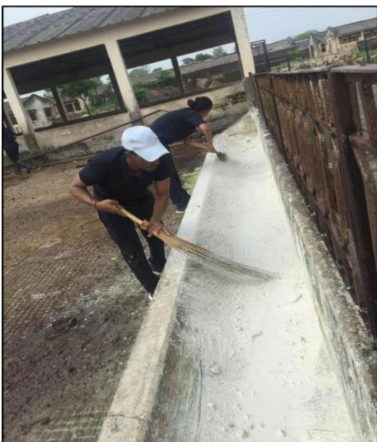
Picture 01- Cleaning and Painting of Waterer at animal shed.
